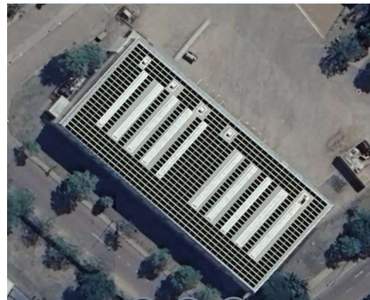
Figure 11 - Roof C2 - 303.05 kWp
