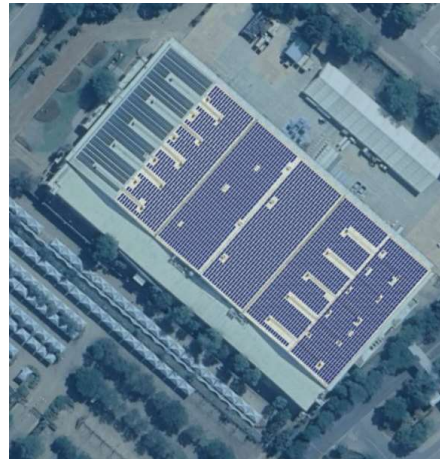
Figure 20 - Roof Yanfeng - 1571.9 kWp
