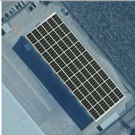
Figure 19 - Roof A11 – 475.2 kWp
