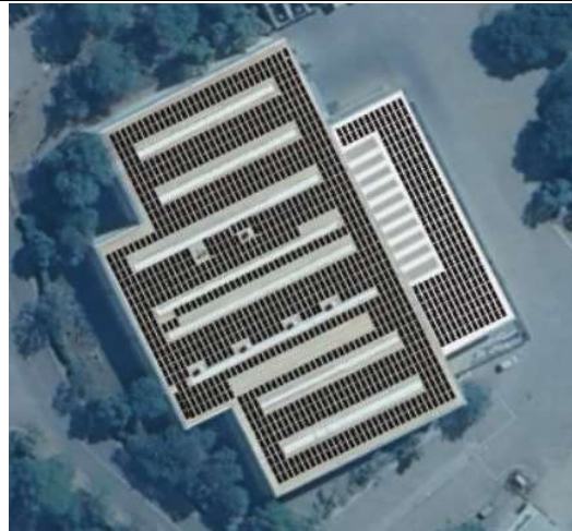
Figure 10 - Roof C1 – 657.7 kWp
