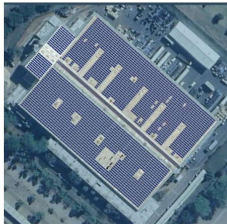
Figure 21 - Roof E4 - 1351 kWp
